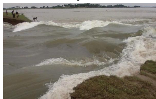
Figure 5.3. Broken embankment in Tahirpur district, Northeast Bangladesh
